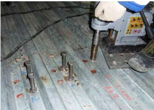
Fig. 10 • Drilling out the sheet for direct welding on the girder.
