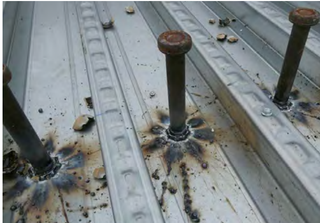
Fig. 13 • Faultlessly through-deck welded studs (Pictures: SLV Munich (4, 5), Trillmich)
