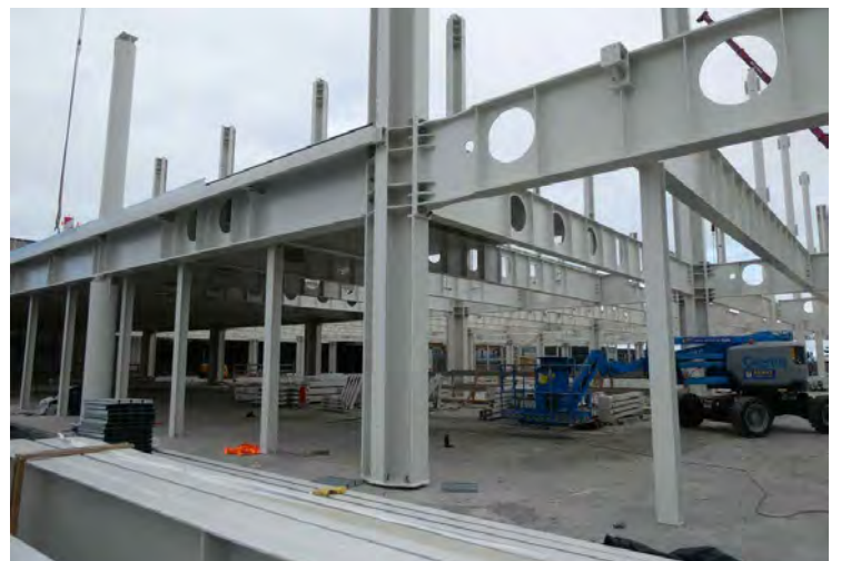
Fig. 12 • Favourable design of the node area for seismic stress absorption.
