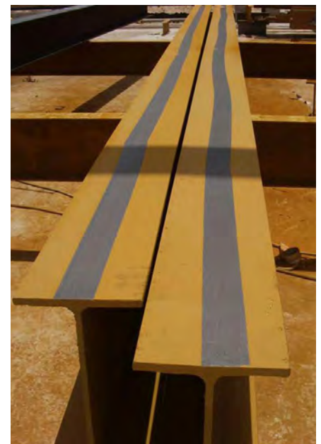
Fig. 7 • The taped area remains without coating.
